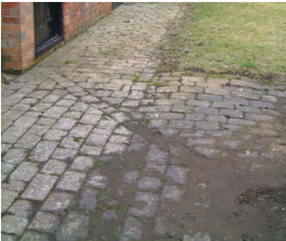
Stable paving. Sarsen stone setts
