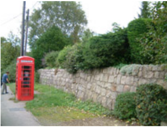
High Street. The telephone call box and a sarsen stone retaining wall
