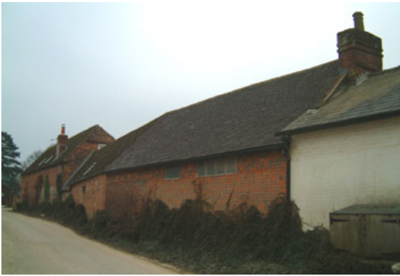
Manton Weir former farm buildings north side
