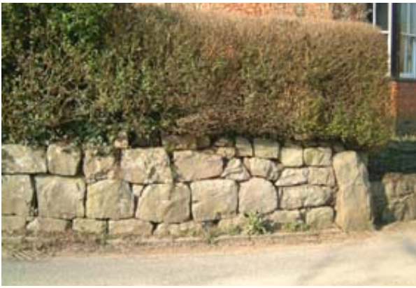
High Street. Sarsen dry stone retaining wall
